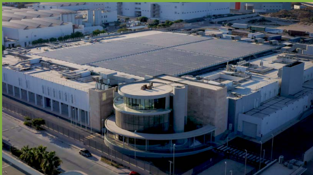
The rooftop solar installation covers an area of over 70,000 square feet.
